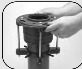
Push drain onto pipe.
